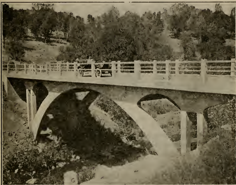
Concrete bridge on the State Highway near Placerville, California.
