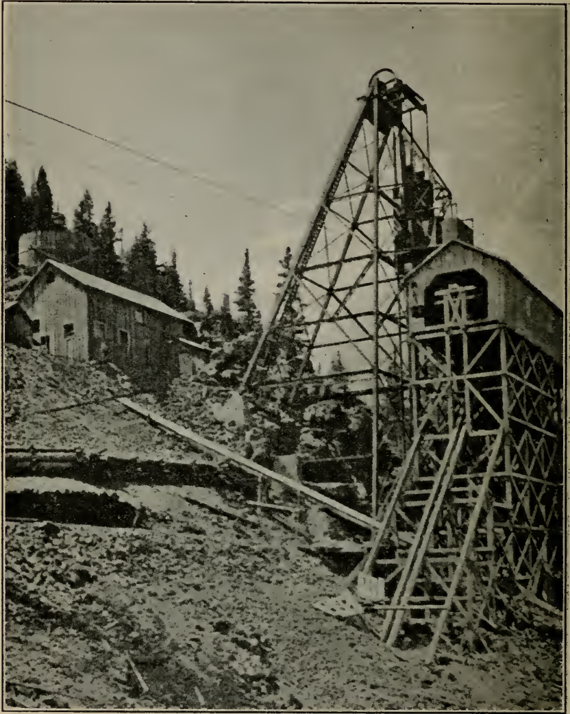
Tramway terminal and head frame at the Superior Mine, Engels Copper Company, Plumas County. Photo by courtesy of the Mining and Scientific Press.
