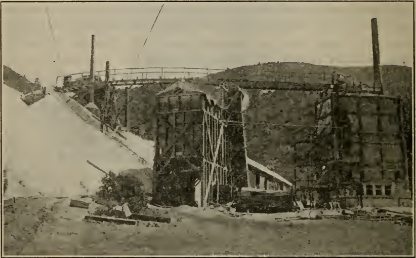
Scott, fine-ore, quicksilver furnace (at right) rebuilt and in use for calcining magnesite fines at Western Magnesite Development Company property, Santa Clara County, Storage bunkers with elevator for calcined fines in center. Four vertical stack kilns at left, for burning lump ore. Photo by courtesy of C. S. Maltby.
