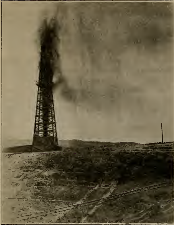
Well flowing over 10,000 barrels of oil per day. Elk Hills, Kern County, California.
