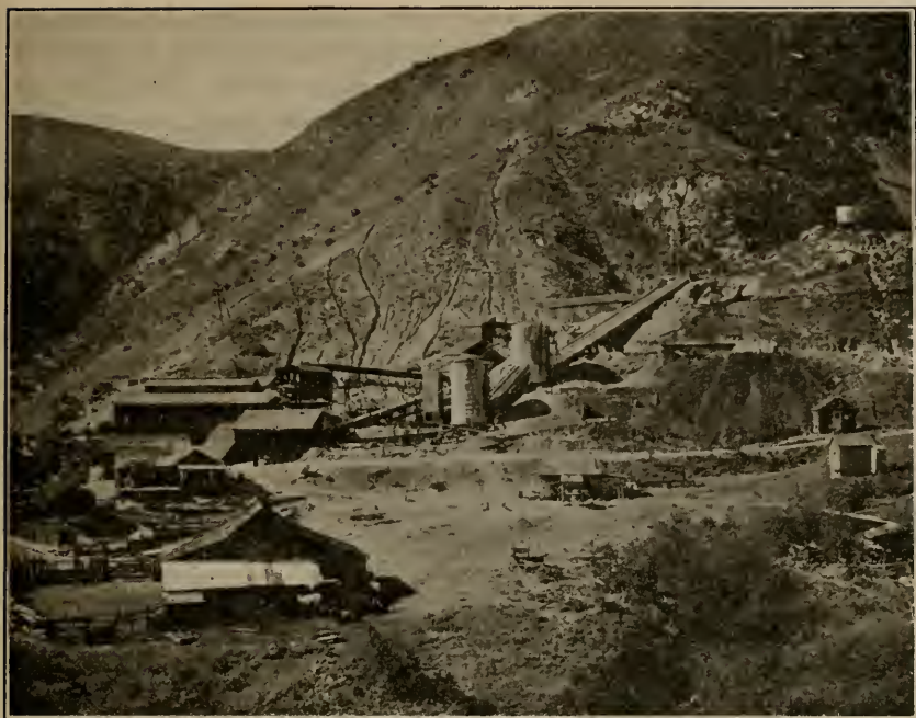
New Idria Quicksilver Mining Company plant, San Benito County, showing reconstruction of condenser system since the fire of June, 1920.
