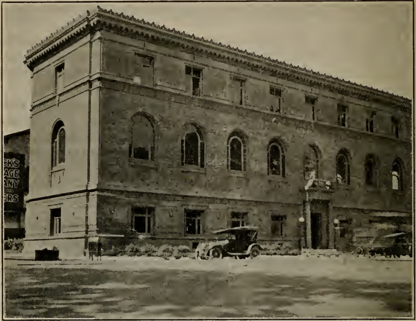
Sacramento City Library, finished with architectural terra cotta and fancy bricks from plant of Gladding-McBean Company, Lincoln, Placer County.
