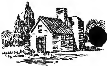
FIG. 3. TOWN SCHOOL AT DEDHAM, MASSACHUSETTS, BUILT IN 1648
