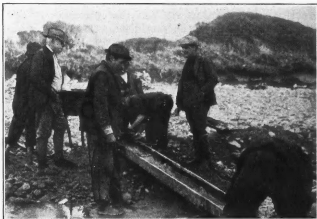
WASHING BEACH SAND. SLUICES LINED WITH BURLAP
