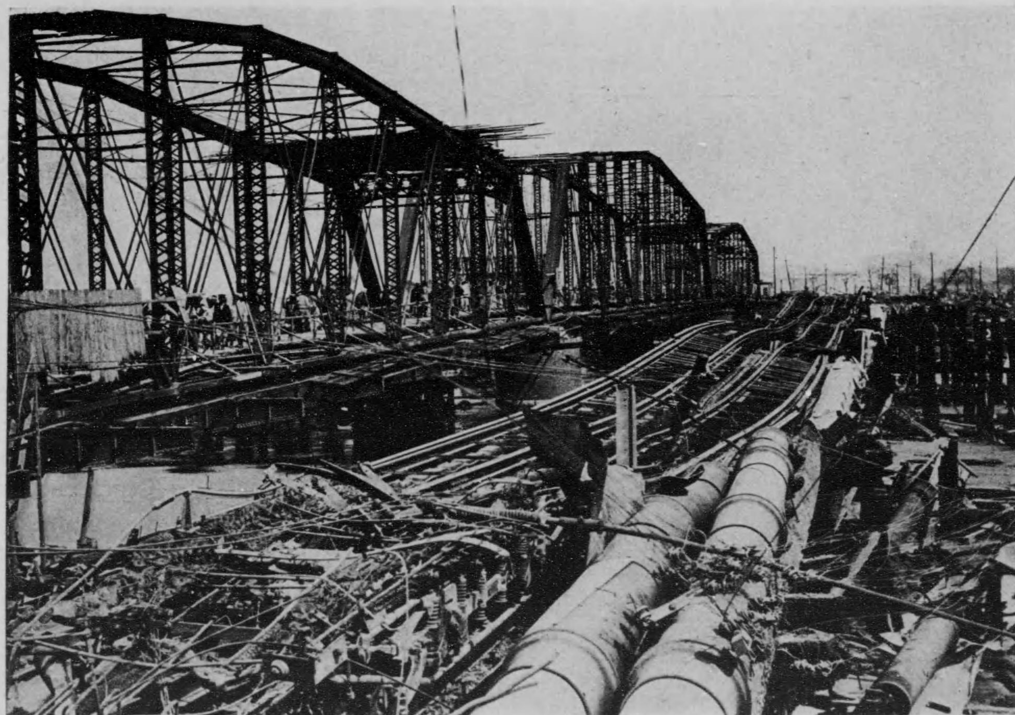
(市京東) 橋代永たし失焼てし残を骨鐵 Famous Eitai Bridge and water mains after earthquake and fire (Tokyo)
