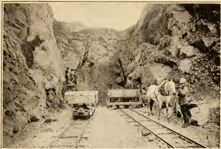
RAILROAD CONSTRUCTION, COPPER RIVER RAILROAD
