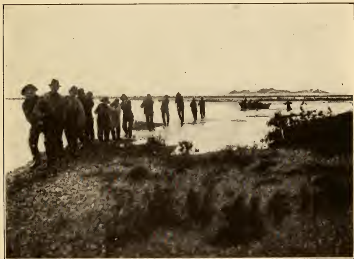
FREIGHTING CONSTRUCTION SUPPLIES UP THE COPPER RIVER
