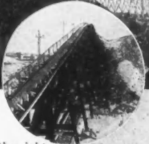
40,000 cords of Pulpwood, Stored and Reclaimed by a Jeffrey Wire Cable Conveyor , 1830 feet centers, at Anglo-New Found-land Development Co.
