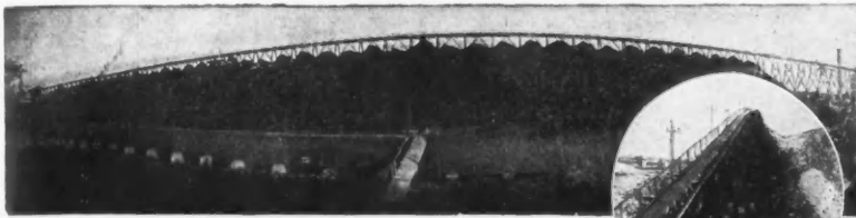
40,000 cords of Pulpwood, Stored and Reclaimed by a Jeffrey Wire Cable Conveyor , 1830 feet centers, at Anglo-New Found-land Development Co.
