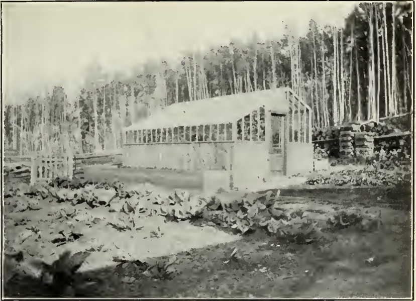
FIG. 1.—NEW PROPAGATING HOUSE, FAIRBANKS STATION.
