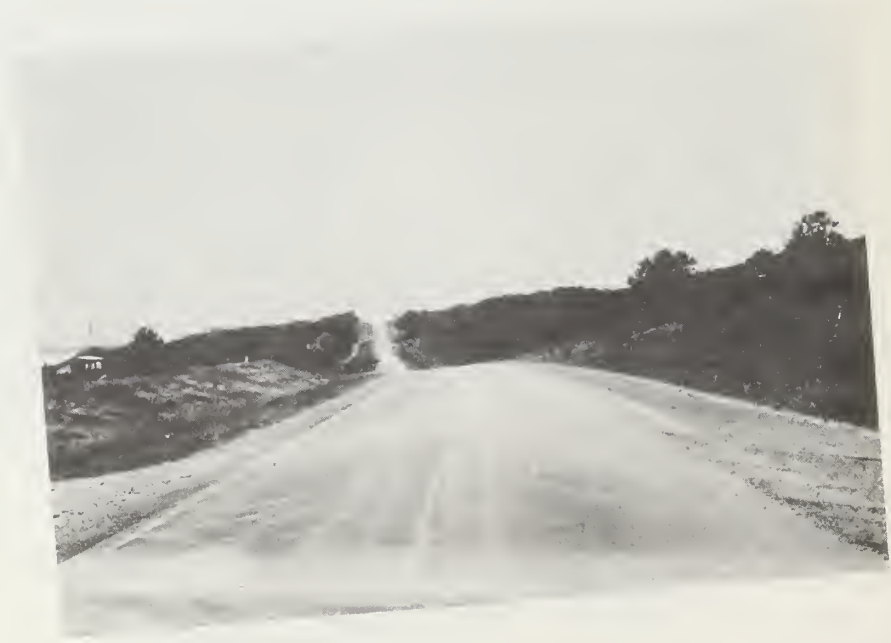
Figure 5. Paved, Marked State Roadway
