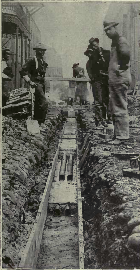
Fig. 586. Laying Fiber Duct
