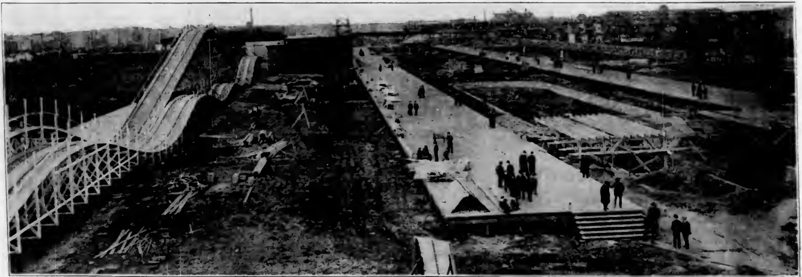
Views Showing How the Work is Progressing at the White City.
