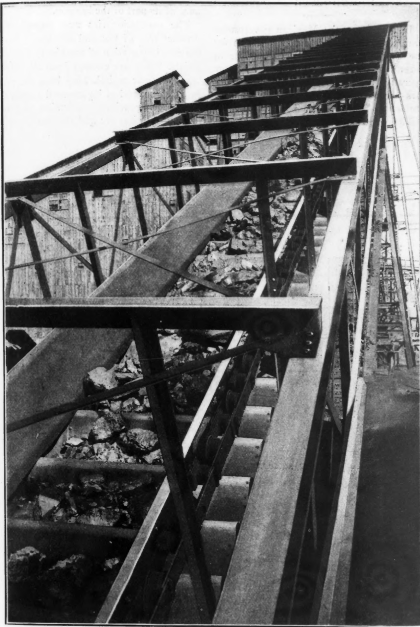
FIG. 6. CARRYING-RUN OF CONVEYER AT PENNSYLVANIA NO. 14 COLLIERY
