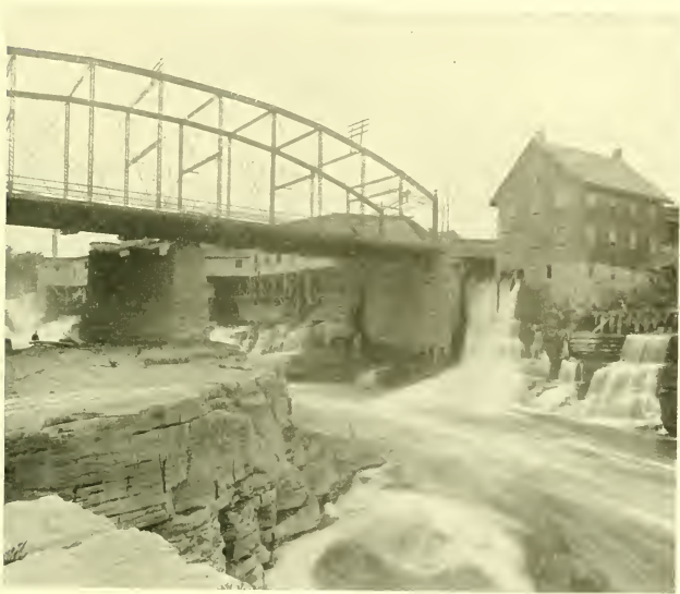
THE BRIDGE AT GLENS FALLS
