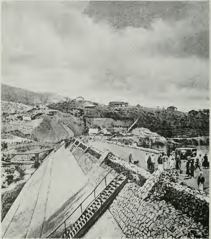
Fig. 71. Periyar dam during construction.
