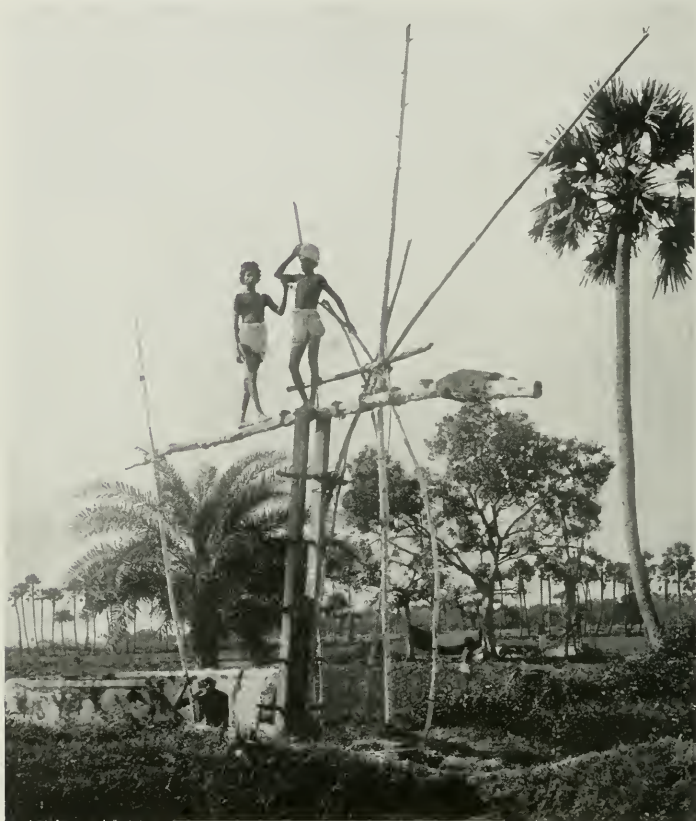
Fig. 70. Lifting water by means of a picota.
