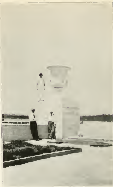
ONE OF THE FOUR MASSIVE GRANITE URNS ON THE PLAZA
