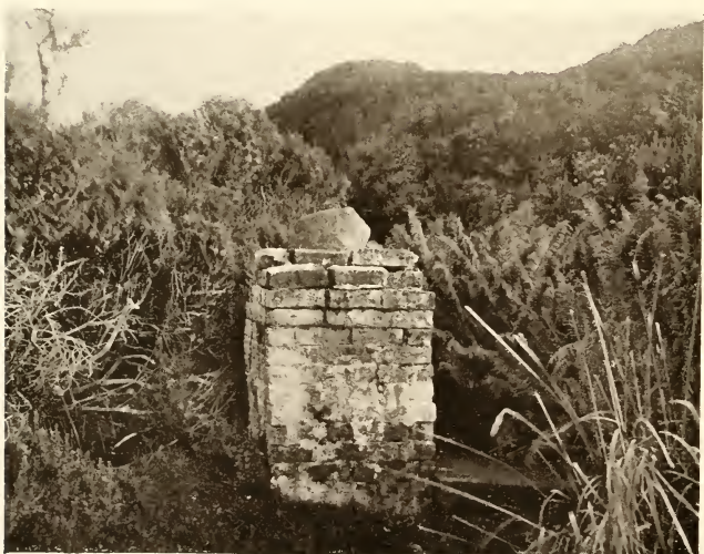
Primmer THE BRICK PIER ERECTED AT PORT ROSS, AUCKLAND ISLANDS, BY THE MAGNETICIANS OF SIR JAMES CLARKE ROSS'S EXPEDITION
