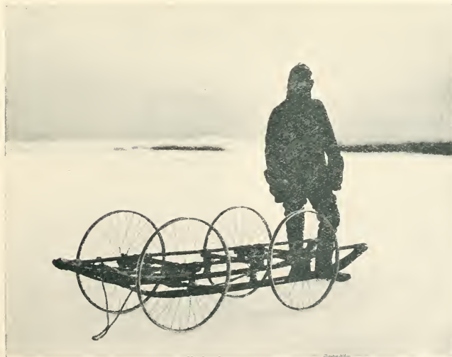
BICKERTON AND HIS SLEDGE WITH DETACHABLE WHEELS
