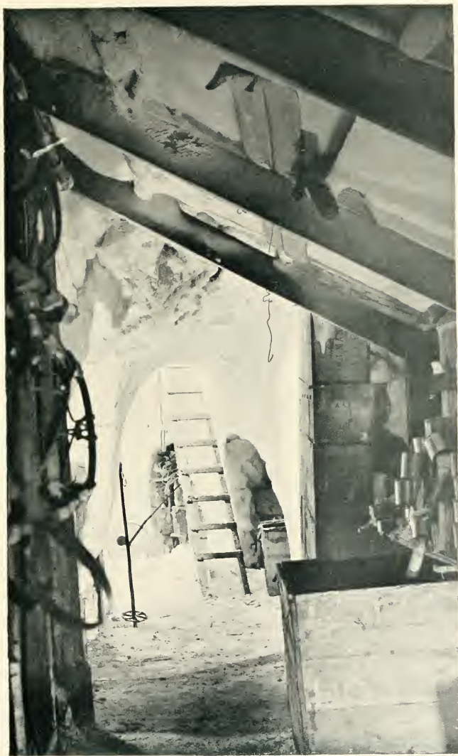
Hoadley IN THE VERANDA OF THE WESTERN BASE HUT—THE GROTTOS—LOOKING TOWARDS THE ENTRANCE DUG VERTICALLY DOWN THROUGH THE SNOW- DRIFT
