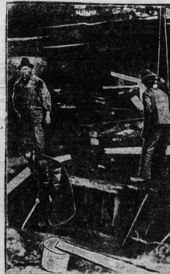
FLOYD COLLINS'S LAST HOPE WHICH FAILED—The shaft sunk in Barren County, Kentucky, in the hope of releasing Floyd Collins from his tomb in Sand Cave is shown above. It is estimated that the tunnel in which Collins was trapped was about sixty feet below the surface. This fact made it necessary to sink a very substantial shaft, heavily timbered.
