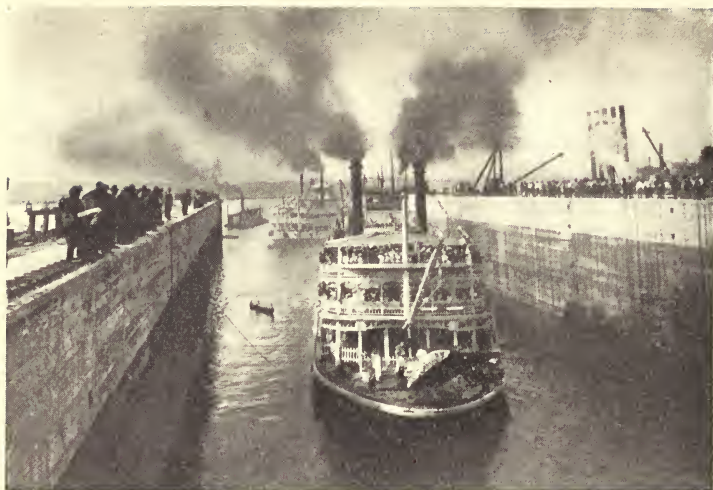
A LOCK AT THE KEOKUK DAM
