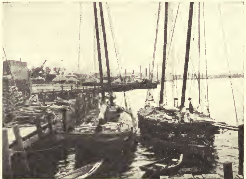
SAILBOATS UNLOADING WOOD AT WHARVES
