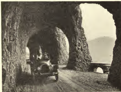
TUNNEL ON COLUMBIA RIVER HIGHWAY
