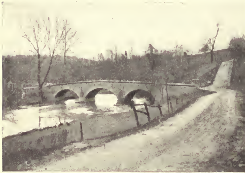
THE BURNSIDE BRIDGE, ANTIETAM BATTLEFIELD
