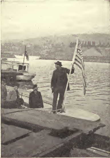
LOOKING ACROSS PORTAGE LAKE TO THE "COPPER PENINSULA"
