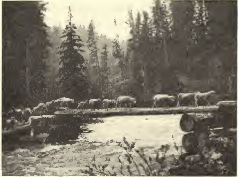
SHEEP BRIDGE ON THE DEADWOOD RIVER
