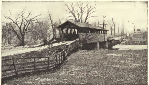
HANGMANS BRIDGE OVER LOST RIVER
