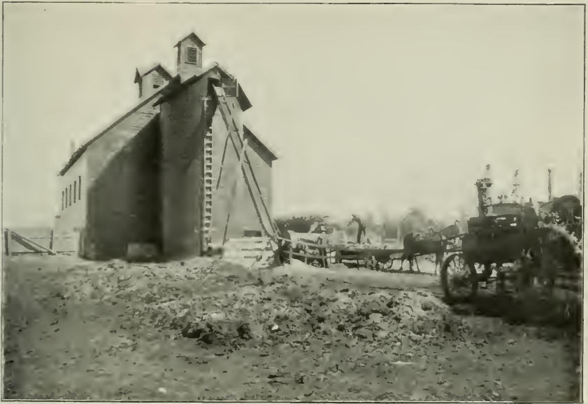
FIG. 1.—A ROUND SILO ATTACHED TO DAIRY BARN ON FARM OF SOUTH DAKOTA AGRICULTURAL COLLEGE, SHOWING METHOD OF FILLING.
