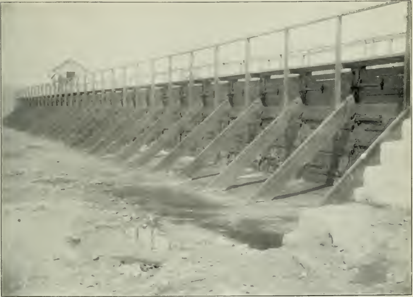
FIG. 1. CANAL WASTE GATE CLOSED.
