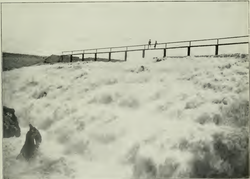
FIG. 2.—CANAL WASTE GATE OPEN.
