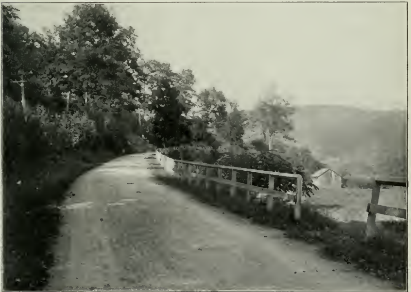
FIG. 2.—TYPE OF ROAD IN MASSACHUSETTS AFTER IMPROVEMENT.
