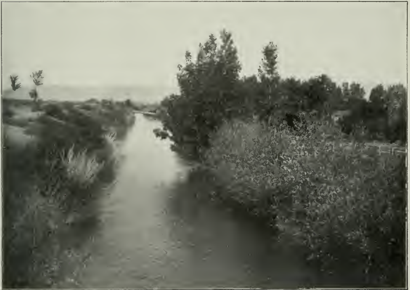
FIG. 2.—APPEARANCE OF IRRIGATION CANAL TEN YEARS AFTER COMPLETION.
