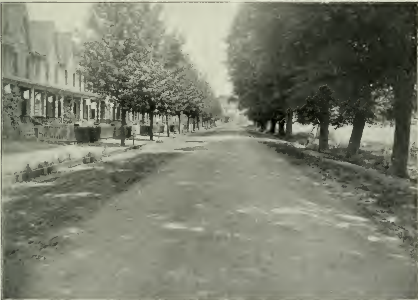
FIG. 2.—TYPE OF ROAD IN NEW JERSEY AFTER IMPROVEMENT.
