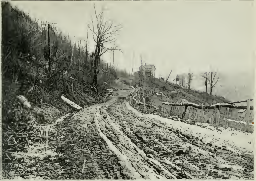
FIG. 1.—TYPE OF ROAD IN MASSACHUSETTS BEFORE IMPROVEMENT.
