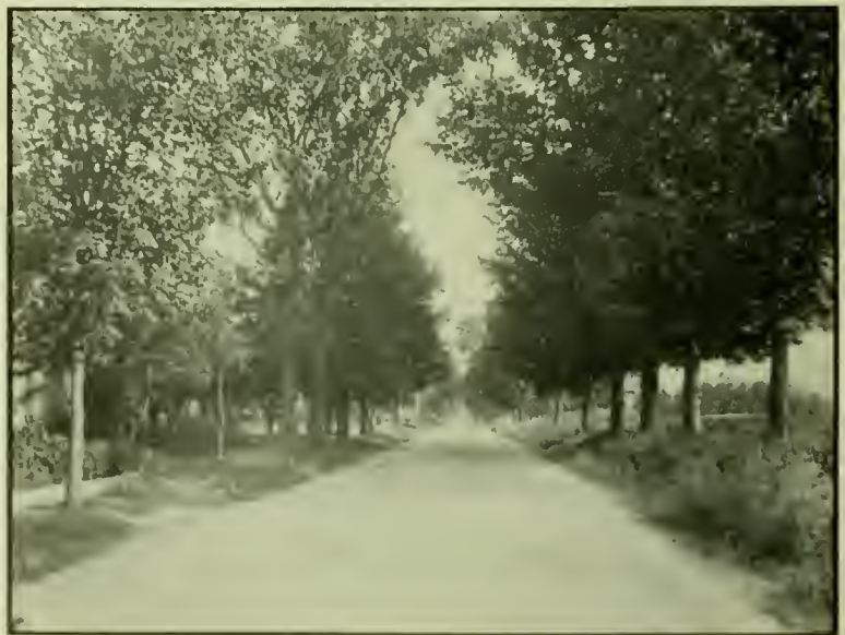
Donwick, Photo. RAILROAD STREET, NORTH FROM CEMETERY STREET.
