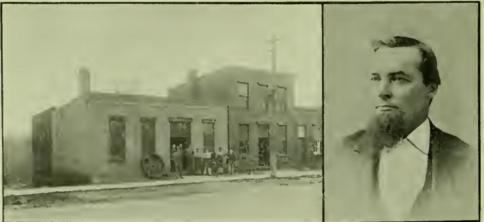
CLARK'S FOUNDRY AND MACHINE SHOP. (Dunwick.)
