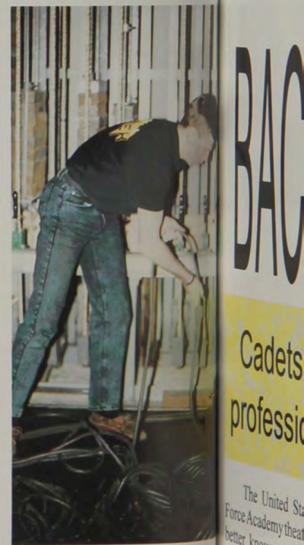
Pulling cable, Mark Hollandsworth makes sure that the cable won't be in the way during the concert. Photo by S. Morris
