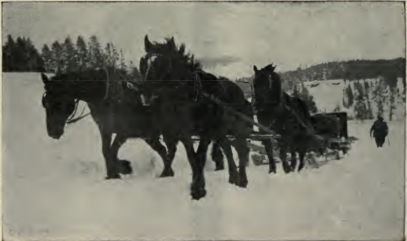
HAULING THE 8,000 POUND GENERATOR
