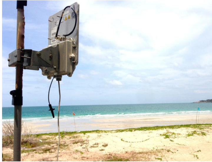
Figure 16. WiMAX Antenna Deployed in Hat Yao, Thailand
