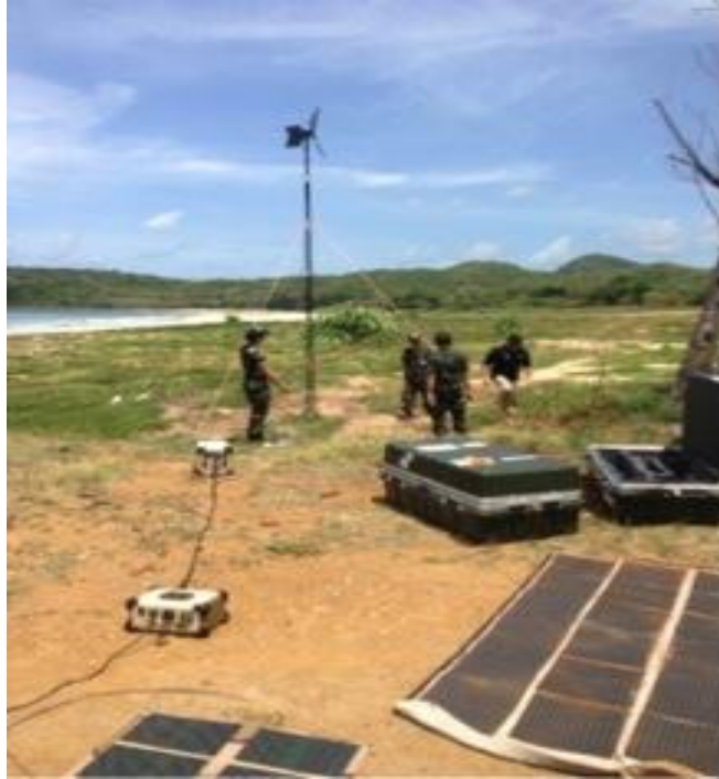
Figure 33. RENEWS Wind Turbine and Solar Panels at Hat Yao Op Area
