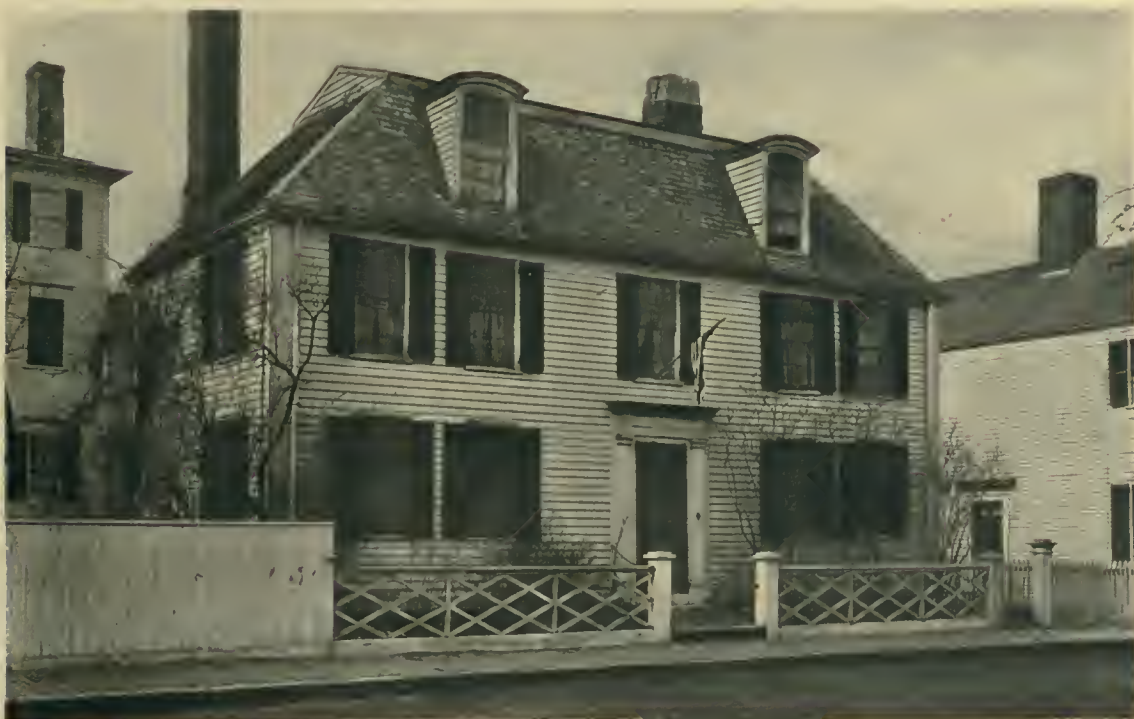
THE FOSTER HOUSE, NEWBURYPORT, MASSACHUSETTS.
