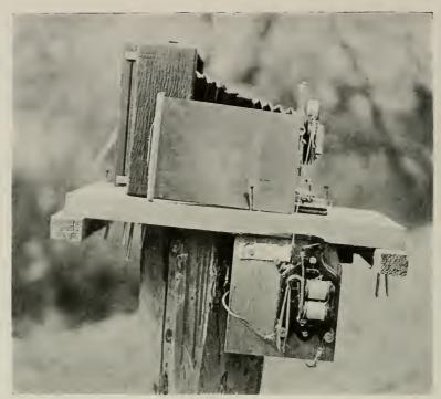
CAMERA SHOWING ATTACHMENT OF ELECTRICAL RELEASE
