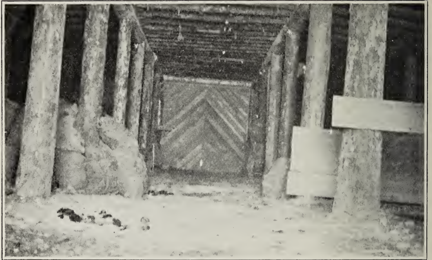
Interior of Potato cellar—round timber construction
