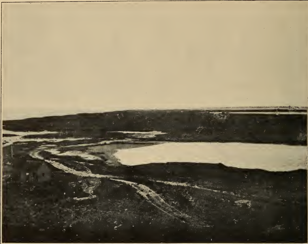
FIGURE 1.—SMITH POINT FROM TOWER OF MADDAKET LIFE SAVING STATION
