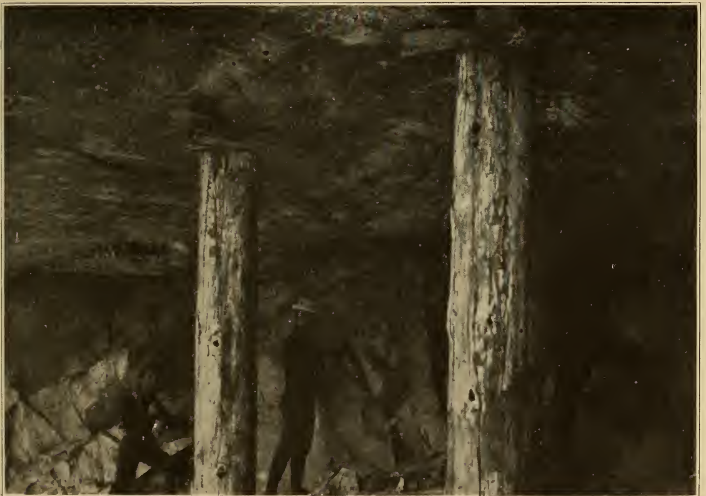
FIGURE 2.—DIP OF QUARTZ VEIN AT FIRST TUNNEL MOLYBDENITE-BEARING VEIN IN GRANITE
