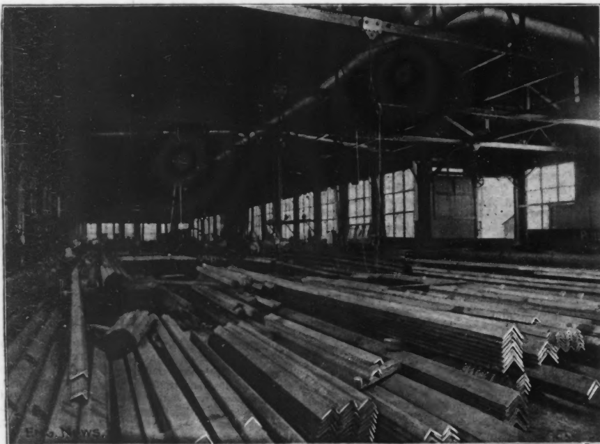
INTERIOR OF MAIN TRUSS SHOP OF THE YOUNGSTOWN BRIDGE CO., SHOWING RAW MATERIAL STORED UNDER COVER.
