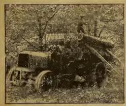
The driver controls the hoisting drum which loads the log
