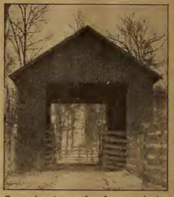
Covered scales are free from weathering and inaccuracies caused by the weather
