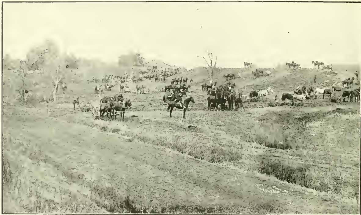
BUILDING LEVEE ON MISSISSIPPI RIVER
