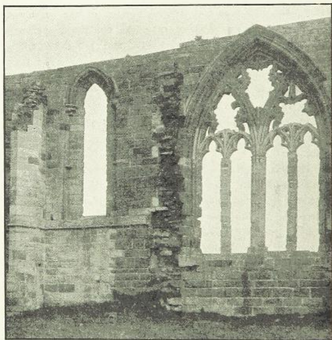
Line of cessation of second building effort—Exterior.
