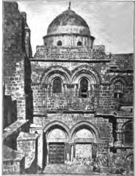
CHURCH OF THE HOLY SEPULCHER Present condition
