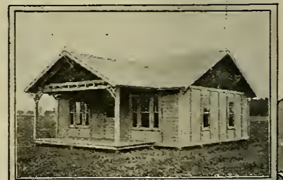
Completed End of Third Day. Ready for occupancy. Two men did it all.
