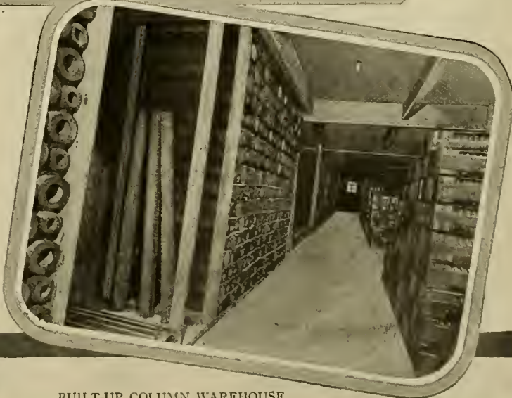
BUILT-UP COLUMN WAREHOUSE
