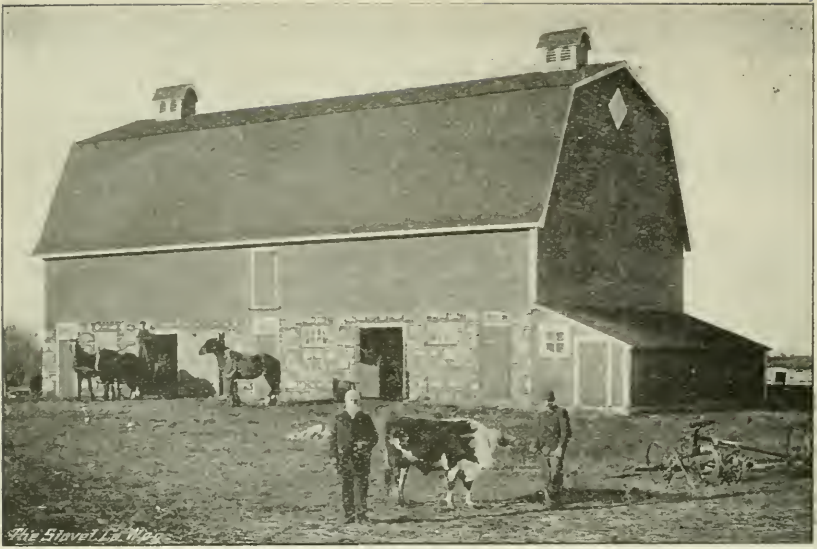
Plank Frame Barn on the farm of F. B. Miller, Solsgirth, Manitoba.
