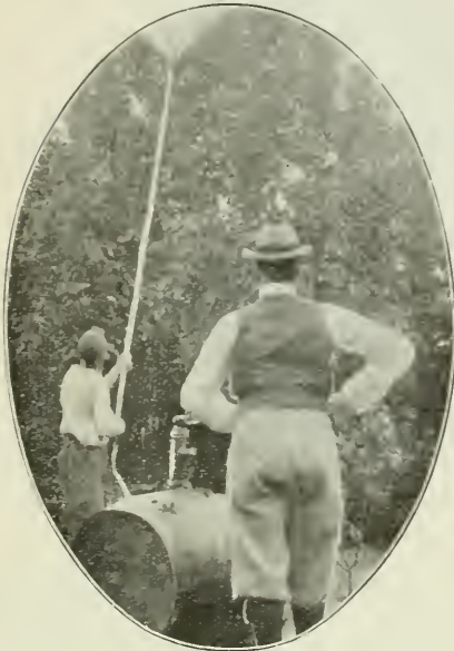
Fig. 7.—Using the bamboo extension rod in spraying young trees.
