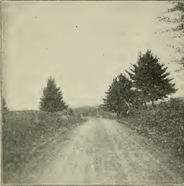
A GRAVEL ROAD IN N. MONAGHAN.—FINISHED IN 1896, AND NOT TOUCHED SINCE.
