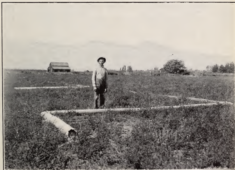
FIG. 2.—DISTRIBUTING WATER FROM SECTIONS OF METAL PIPE ATTACHED TO MAIN PIPE BY CANVAS ELBOWS.
