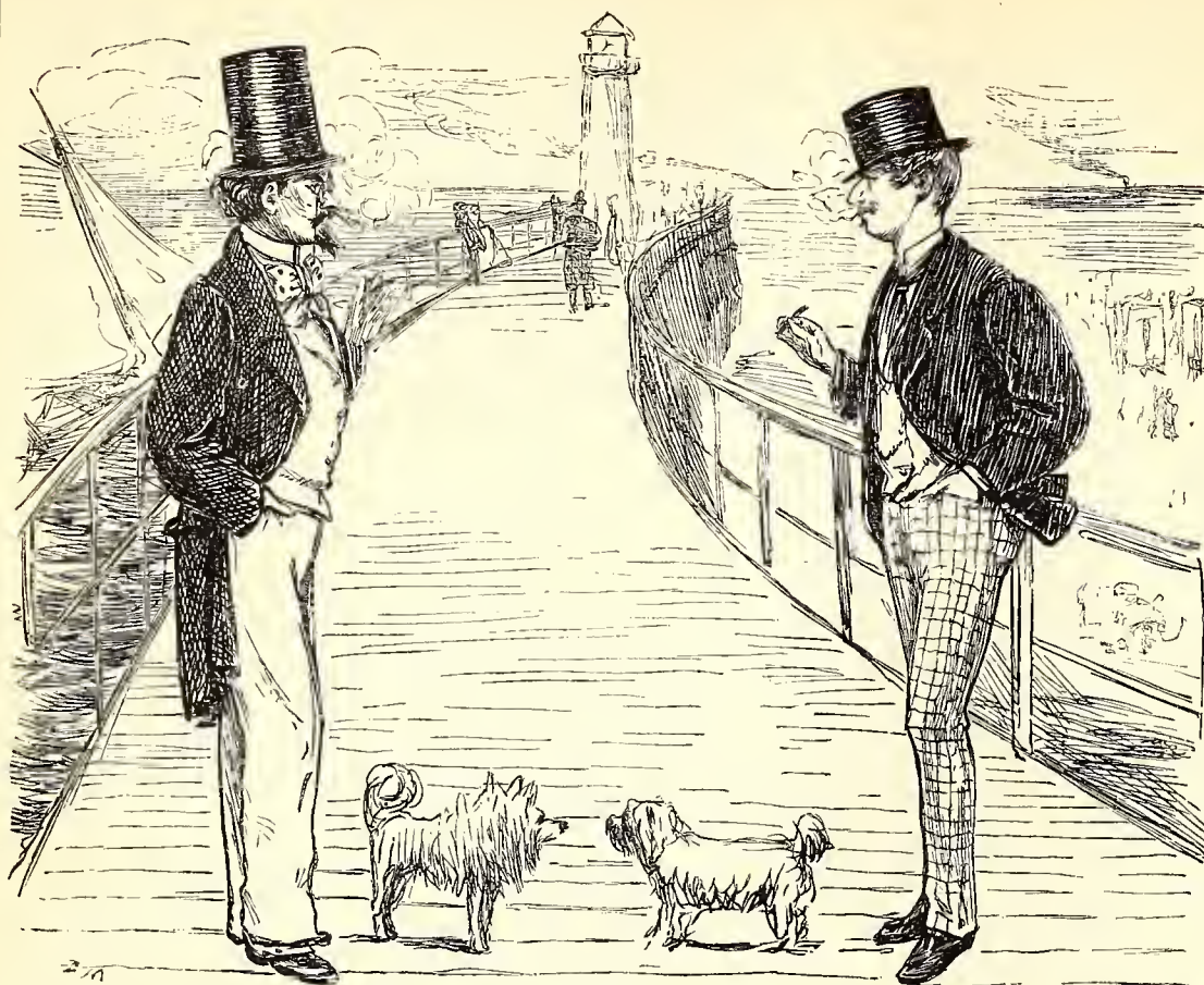
ON THE BOULOGNE PIER.
