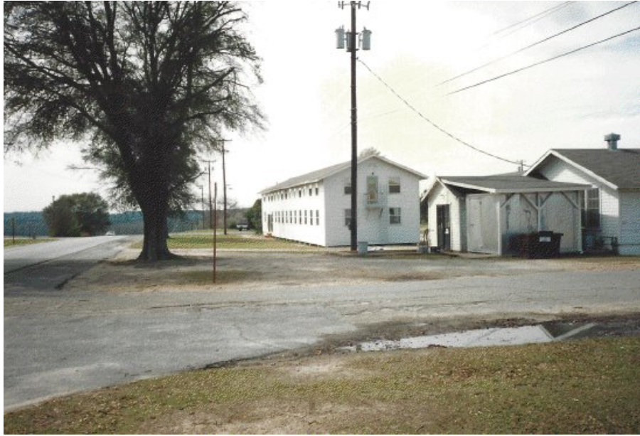
Figure 19. RIP Barracks and RTD Chow Hall in 1984 319
