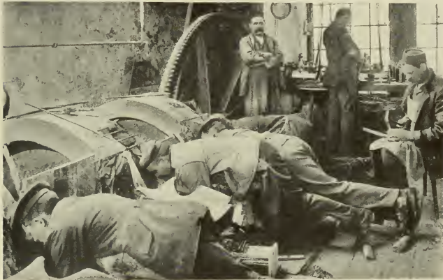
FIG. 29.—Grinding agates. Oberstein—Idar.
