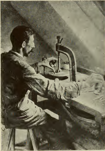
FIG. 32.—Grinding facets on gem stone.
