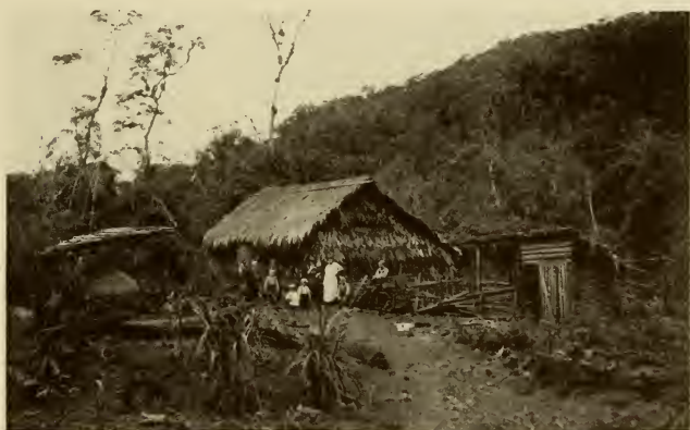
FIG. 46.—House in Blumenau similar to the one which formed the early home of Fritz Müller.
