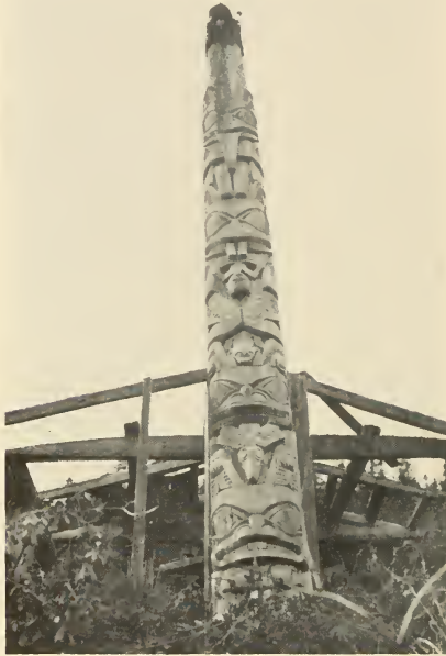
FIG. 178.—Frame and roof timbers of Eagle House "hut-nes" with "Eagle King's" totem pole at the front. This house is the sole remaining structure at Old Kasaan, and with the house of Jim Peel at New Kasaan, is the only surviving native house in southern southeast Alaska. Crests on pole are: eagle, at top; beaver, at bottom; bear, with protruding tongue, beaver, with large projecting upper incisor teeth, and figures illustrating the myth of "Raven Traveling," at center. See fig. 177.
