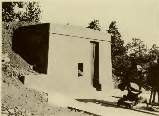
FIG. 32.—Concrete observing tunnel at Table Mountain, California.
