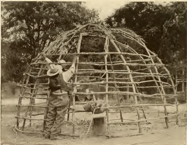
FIG. 108.—Framework of wigwam of Southern Californian Indians; constructed under Mr. Harrington's direction.
