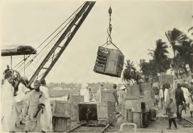
FIG. 25.—Handling stock at Dar-es-Salaam.
