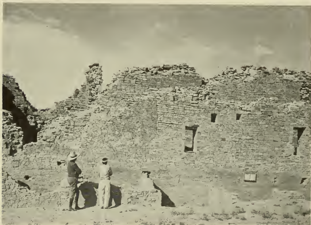
FIG. 166.—Outer south wall of Pueblo del Arroyo, showing varied stonework and later, abutting rooms. (Photograph by Neil M. Judd. Courtesy of the National Geographic Society.)
