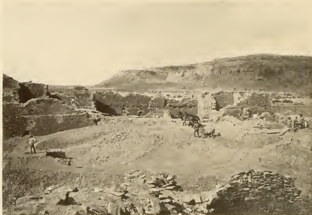
FIG. 88.—In excavating the central portion of Pueblo del Arroyo, debris from the individual rooms was wheeled in barrows to accessible points and dragged thence to an elevated trap through which it was poured into steel tram cars. (Photograph by O. C. Havens. Courtesy of the National Geographic Society.)
