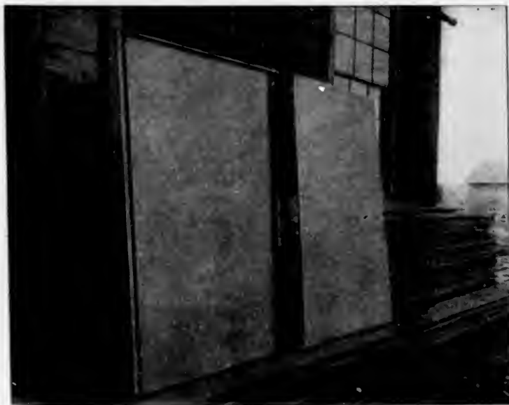
Rear View of the Ruby Sectional Steel Sign showing steel braces and galvanized sections in place.
