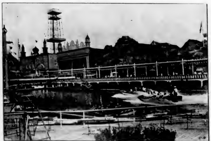
Bottom of the Chutes.
