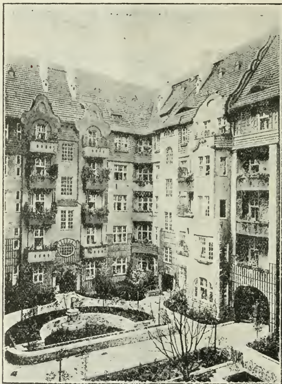
WORKING MEN'S FLATS AT RIXDORFER STRASSE, BERLIN.
