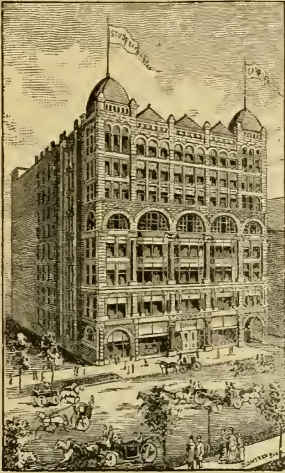
THE STUDEBAKER BUILDING, MICHIGAN AVENUE BETWEEN VAN BUREN AND CONGRESS STREETS.
