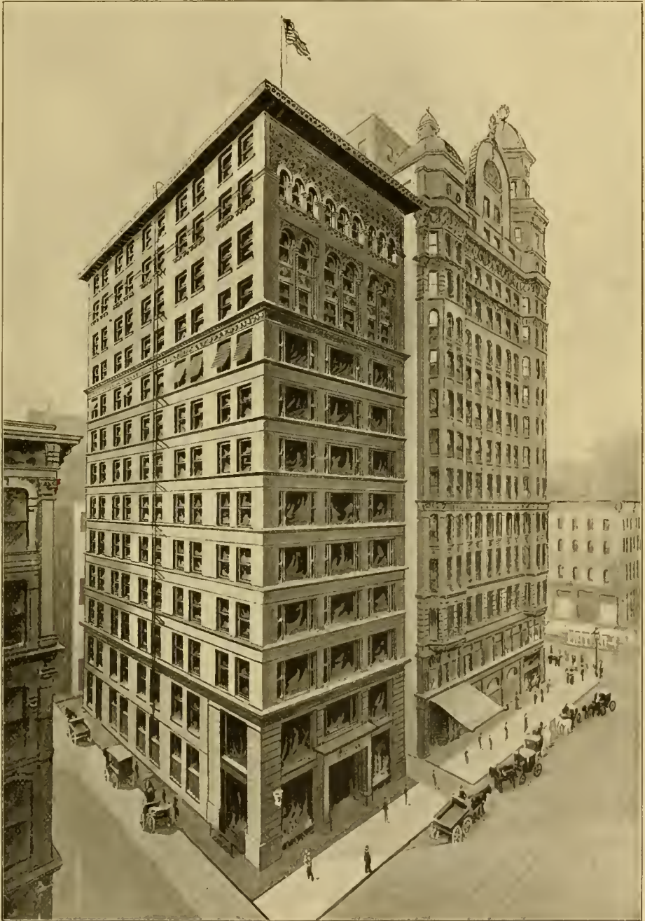
THE VENETIAN BUILDING. 34-36 WASHINGTON STREET, BETWEEN STATE STREET AND WABASH AVENUE.
