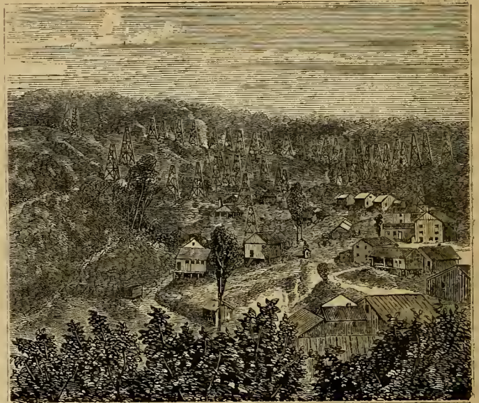
PLEASANTVILLE.—VIEW OF THE DERRICKS.
