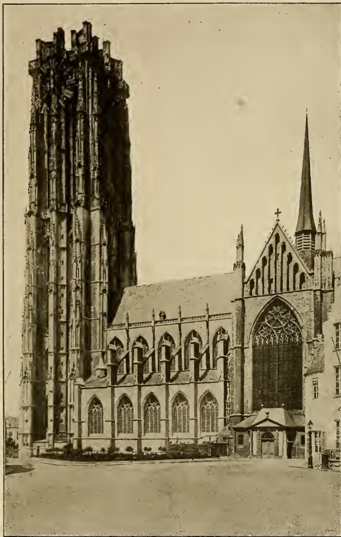
CATHEDRAL OF ST. ROMBAUT. MALINES.
