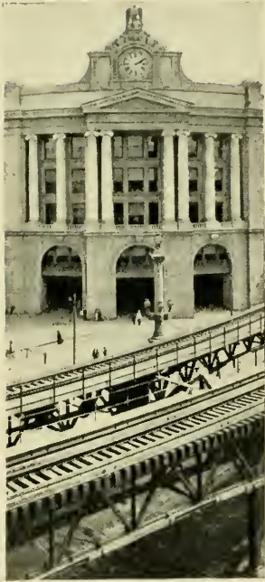
ENTRANCE TO SOUTH TERMINAL STATION.
