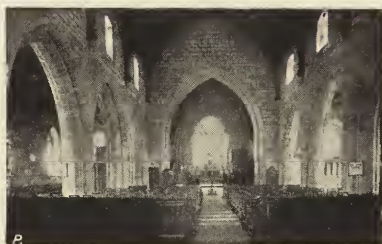
NAVE, LOOKING EAST.
