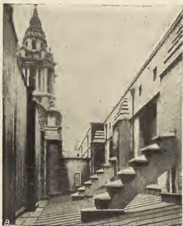
FLYING-BUTTRESSES AND SCREEN-WALL.
