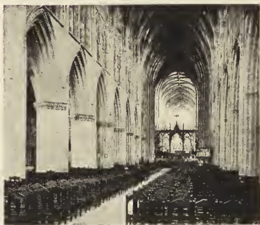
NAVE, LOOKING EAST.
