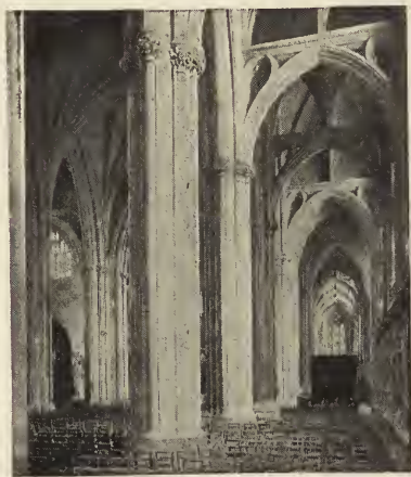
VAULT OF AISLE.
