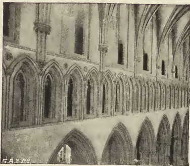
TRIFORIUM OF NAVE.
