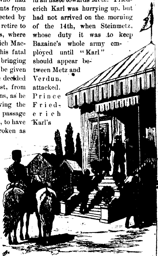
HEAD-QUARTERS OF NAPOLEON AT CHÂLONS.
