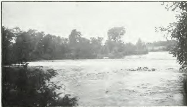
No. 51.—Dam at St. Andrews, Quebec, on the North River.
