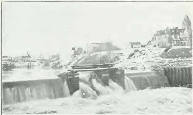
No. 29.—Indian River dam at Pembroke, showing ordinary high water flow.
