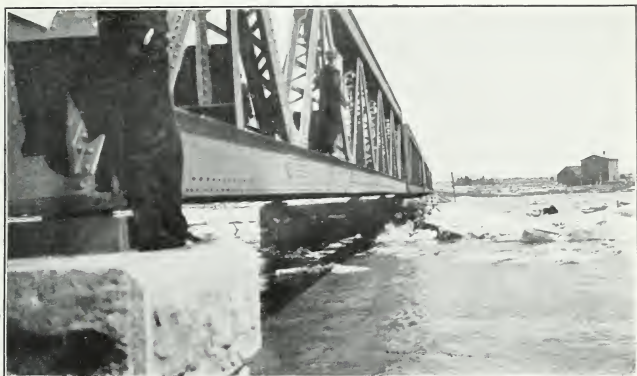
No. 47.—South Nation River C. P. R. bridge, utilized as a metering and gaging station for this part of the river.
