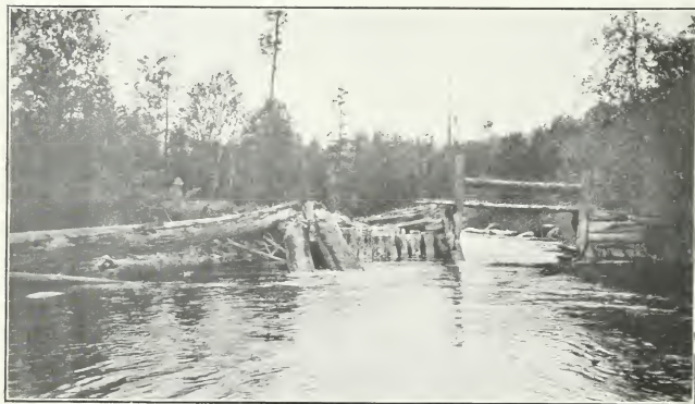
No. 72.—Log chute in Lumberman's dam at outlet of Rock Lake.
