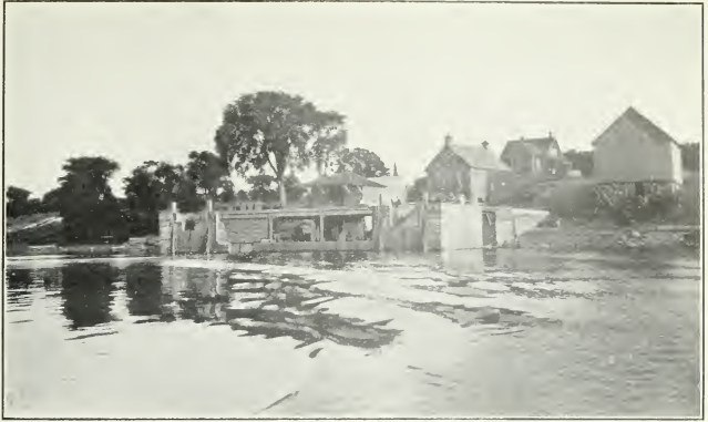
Cumberland, Ont. Double deck cribwork wharf.
