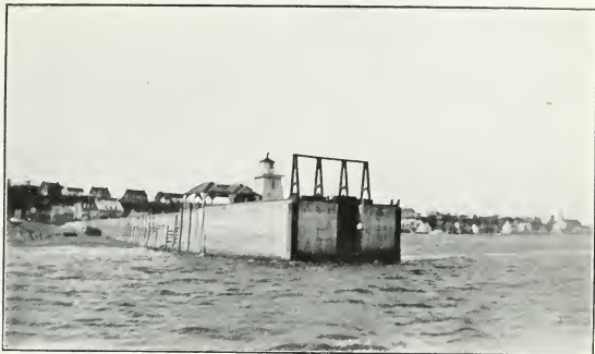
St. Jean (Island of Orleans), P.Q., close faced pilework.
