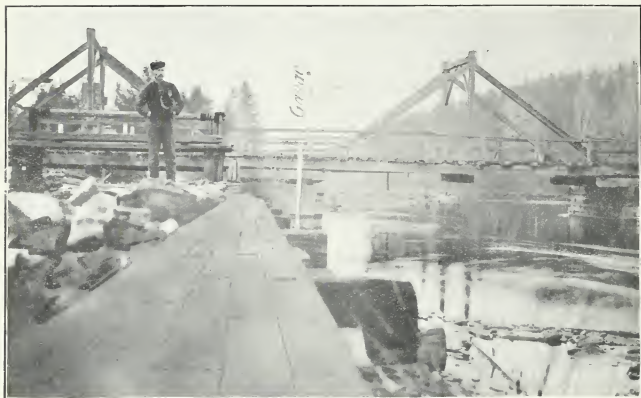
No. 24.—Black River gaging and metering station at Waltham, Quebec.
