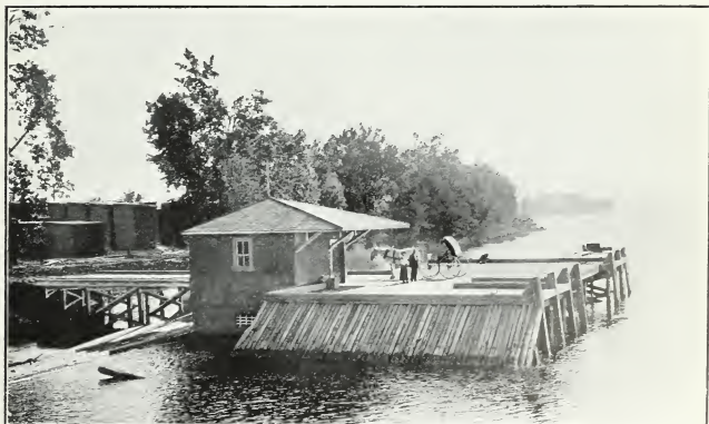
East Templeton, P.Q., pilework wharf.
