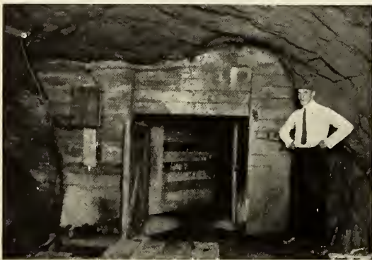
THE DOORWAY LEADING INTO THE DYNAMITE MAGAZINE.
