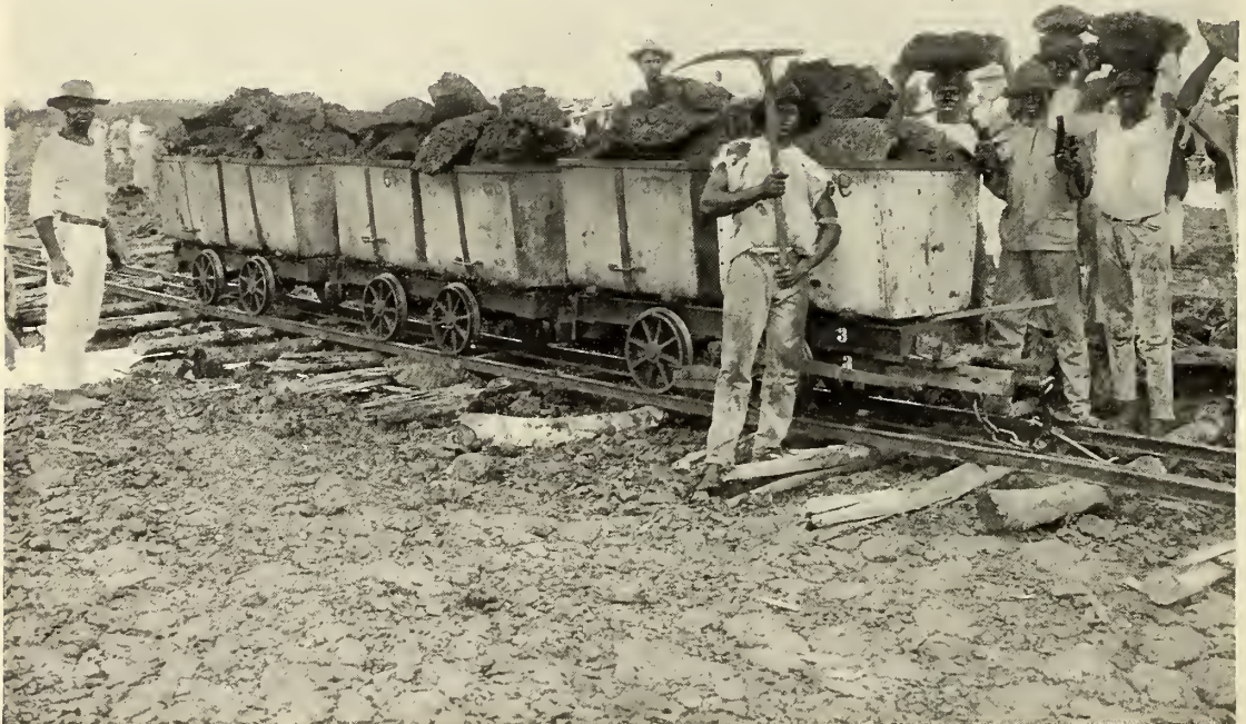
LOADING CARS WITH ASPHALT.
