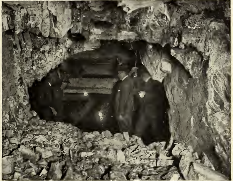
"HOLED THROUGH." THE JUNCTION OF TWO TUNNEL HEADINGS.
