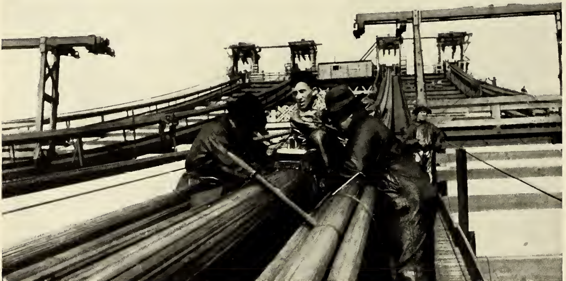
"SEVERAL STRANDS WERE SQUEEZED TOGETHER TO FORM A CORE." (SEE PAGE 740.)
