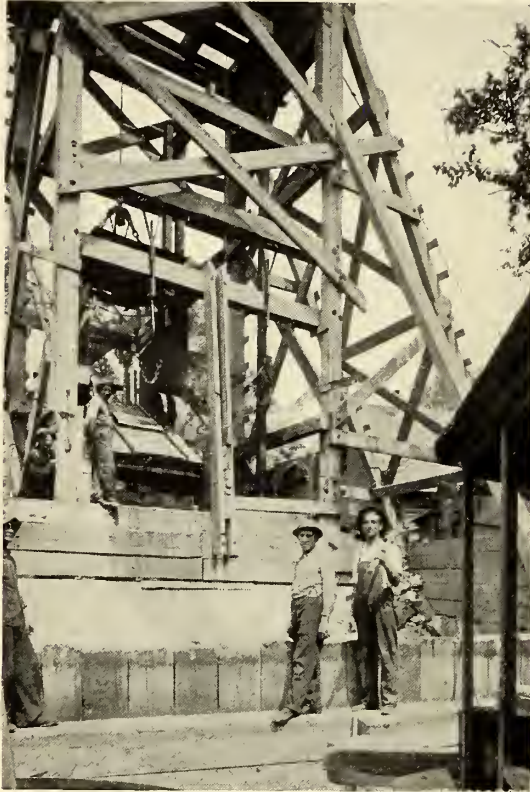
THE HEAD-FRAME OF AN AQUEDUCT SHAFT IN CENTRAL PARK, NEW YORK CITY.
