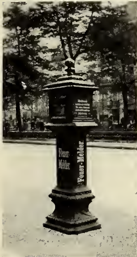
A BERLIN FIRE-ALARM BOX.
