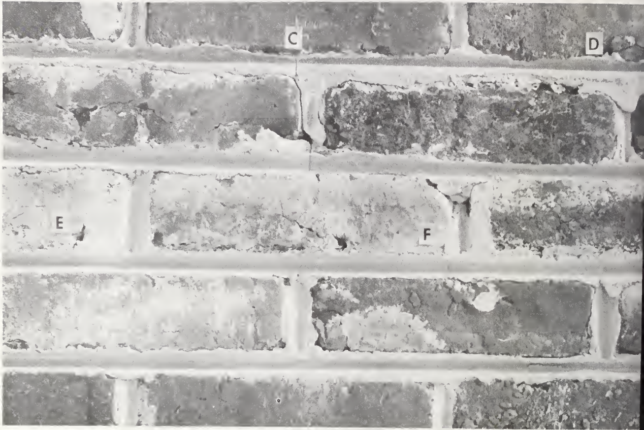
Figure 2. Section of a Clay Brick Wall Exhibiting Several Types of Openings.
