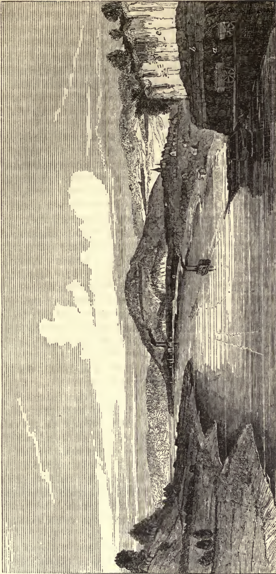
View of the great Coal Seam on the Monongahela at Brownsville, Pennsylvania, U. S. b. Black bituminous or carbonaceous shale, 10 feet thick. d d. Upper seam of coal, 6 feet thick.
