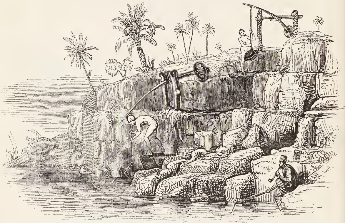
B. Modern shadóof , or pole and bucket, used for raising water, in Upper and Lower Egypt.
